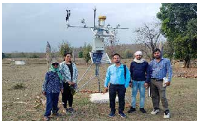
Installation of AWS at Kanha Tiger Researve
